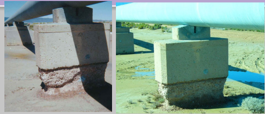
Damage stops at capillary break at interface of foundation with support concrete
