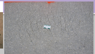
Tearing of Bridge Deck Surface due to premature loss of workability
