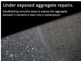
Under exposed aggregate repairs. Sandblasting concrete away to expose the aggregate beneath it converts a mess into a masterpiece!
