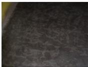
Non Breathable Membrane placed over fresh concrete trapped moisture creating spotting or "leopard" pattern.
