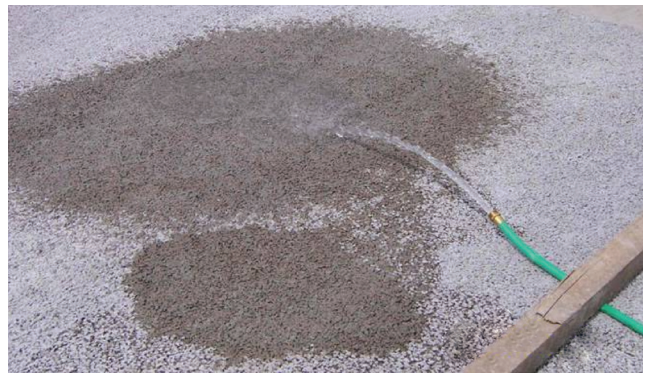
Figure 9.2 Pervious concrete (photo courtesy of John KeVERN, University of Missouri-Kansas City)
