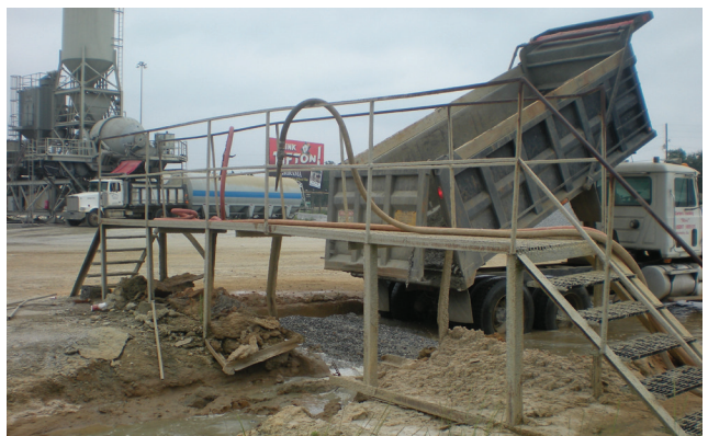
Figure 5.8 Washout pit used to clean concrete trucks (photo courtesy of Gary Fick, Trinity Construction Management, Inc.)
