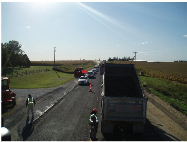
Figure 6.5 Traffic delays caused by construction (photo courtesy of Jim Cable, FHWA)
