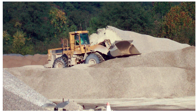
Figure 5.2 Front-end loader used for stockpiling aggregate (photo courtesy of Gary Fick, Trinity Construction Management, Inc.)
