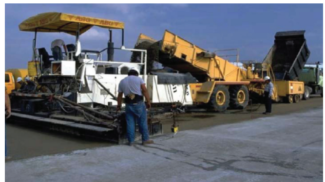
Figure 5.14 RCC placement (Harrington et al. 2010)
