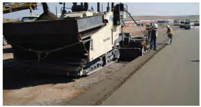
Figure 3.4 RCC pavement being placed (photo courtesy of PCA)
