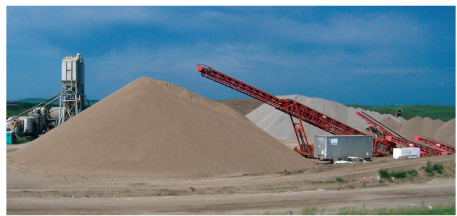
Figure 5.3 Stockpiling aggregate with a radial stacker (photo courtesy of Gary Fick, Trinity Construction Management, Inc.)
