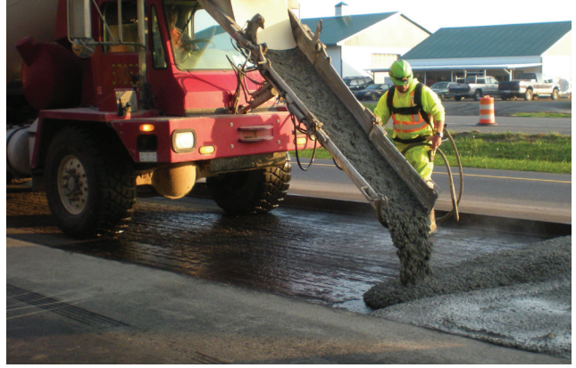
Figure 5.6 Transit mix concrete truck (photo courtesy of Gary Fick, Trinity Construction Management, Inc.)
