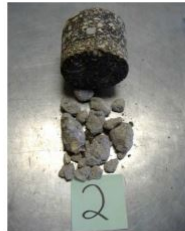
Figure 7. Typical core of asphalt parking lot with granular subbase
