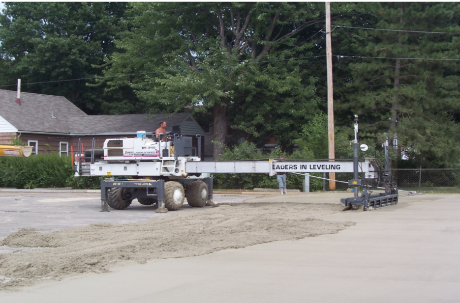
Laser guided screed
