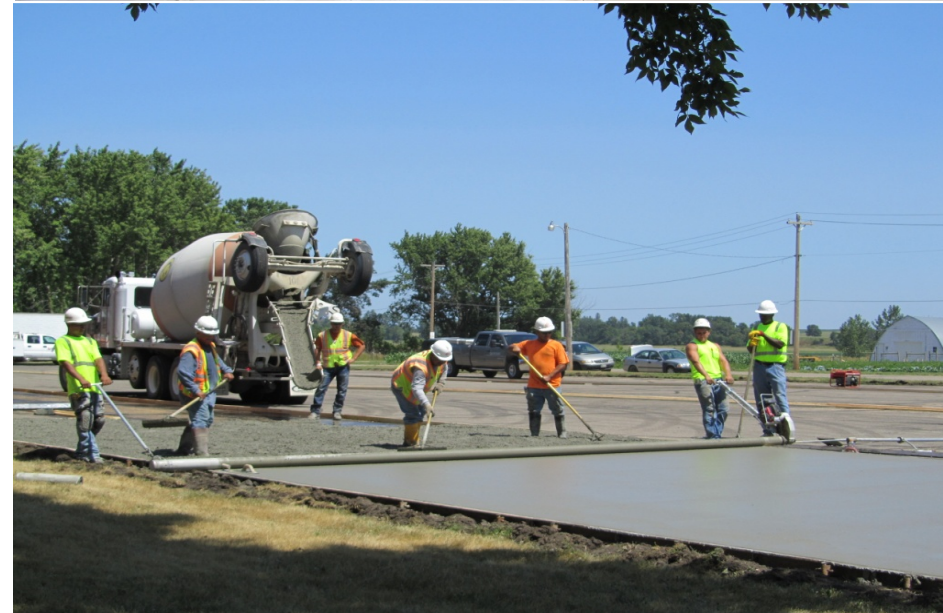
Spinning roller screed
