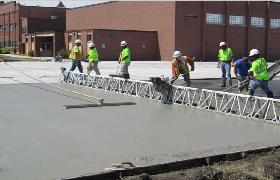
Truss frame screed
