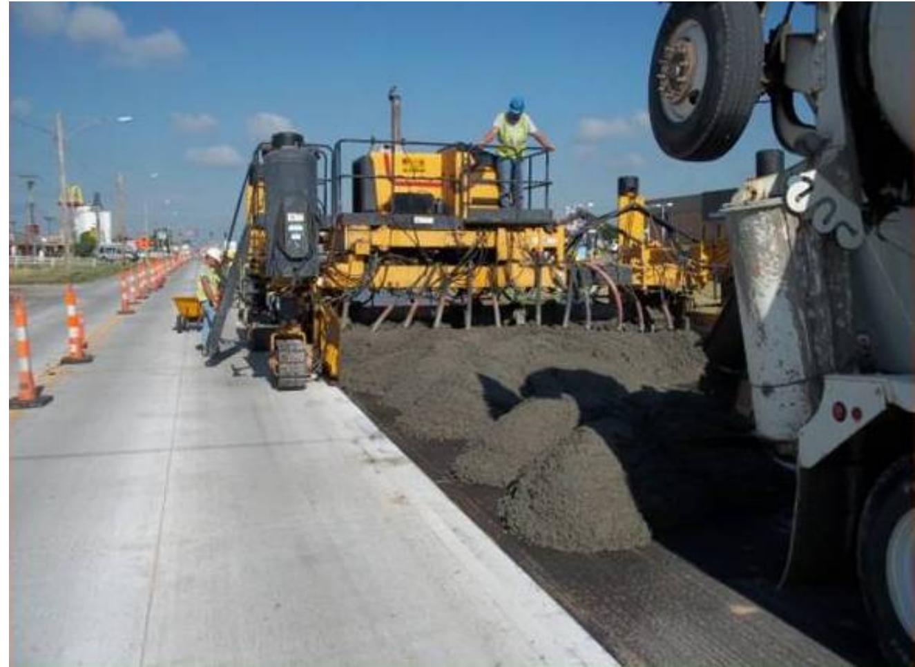
Slipform paver placement
