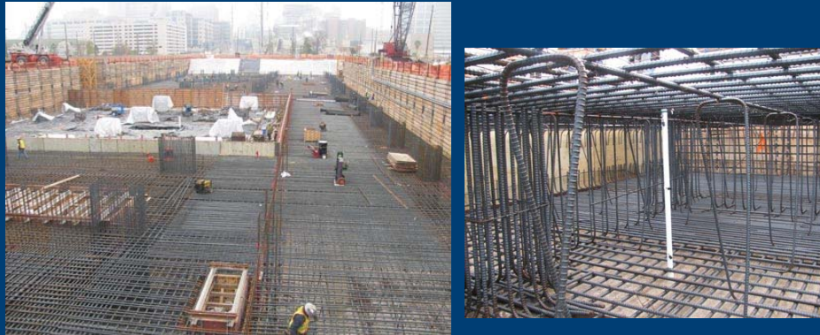
Mat foundation, courtesy of Carrasquillo Associates
