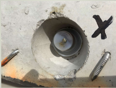
Note steel puncture in cap
