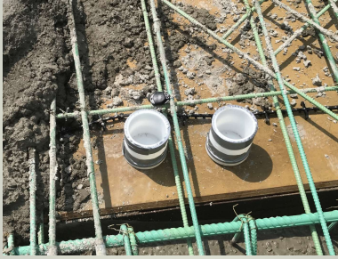
Cast in place punch out cylincores (CIPPOC's). With probe
