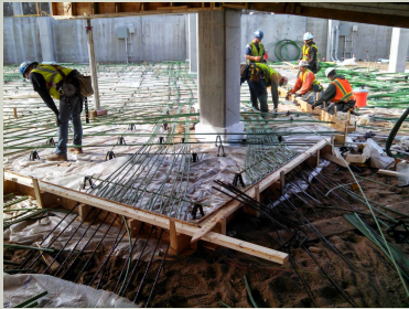
Note drape, sweep, and bulkheads
