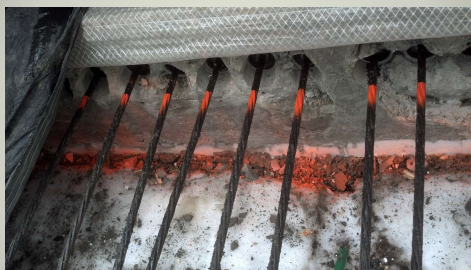
Marking tendons prior to stressing
