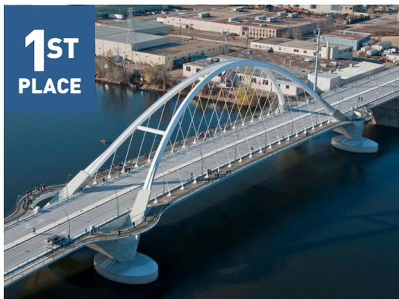
**Lowry Avenue Bridge.** The 80 million dollar Basket handle tied-arch bridge construction started in early 2010 and opened for traffic October 27, 2012. Total Cost \$104 million. 1,576 foot long, 107 feet wide. 10,820 yd<sup>3</sup> of concrete was used in this project.
