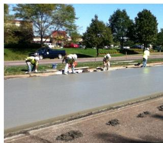
**CP 12-11601 Asphalt Mill and Concrete Overlay: Valley Creek Road from Bielenberg Drive to Woodbury Drive.** Aggregate Industries supplied approximately 10,000 yd<sup>3</sup> of concrete for a 1.5 mile unbonded overlay on Valley Creek Drive in Woodbury, MN which included high early concrete to accelerate intersection openings.
