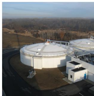
**Blue Lake Waste Water Treatment Plant.** Cast-in-place concrete is ideal for corrosive environments such as waste water treatment plants because of its durability, flexibility and functionality.
