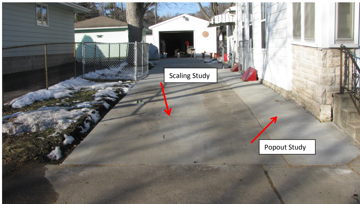
Photo 1: Overall view of research slabs.
