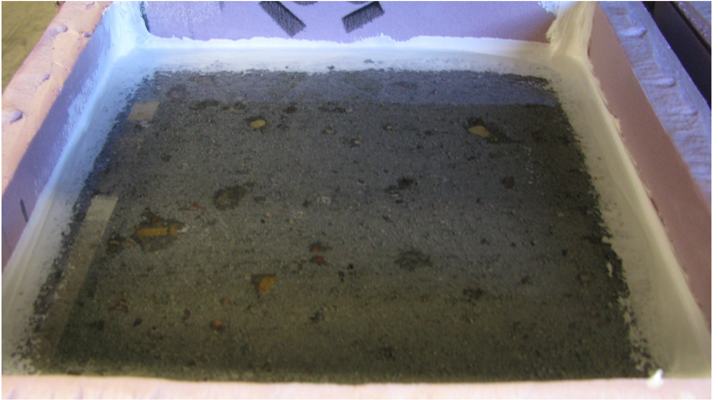
Photo 3: Showing scaling of ASTM C672 panel #7 after 50 cycles.
