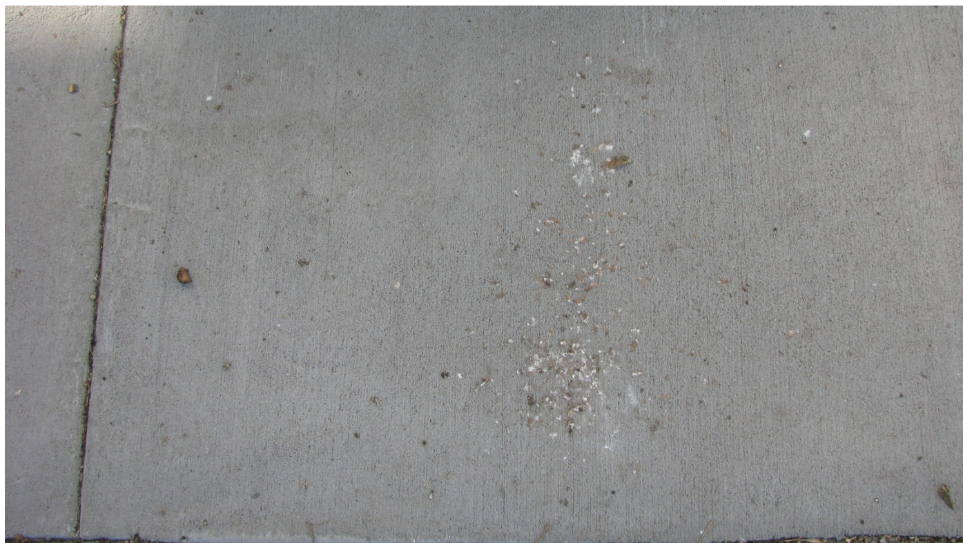
Photo 2: Showing initial popouts in slab #7 of the popout study.
