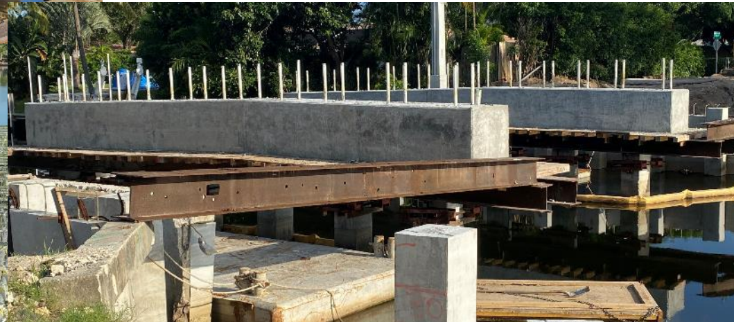
Casting completed and forms stripped
