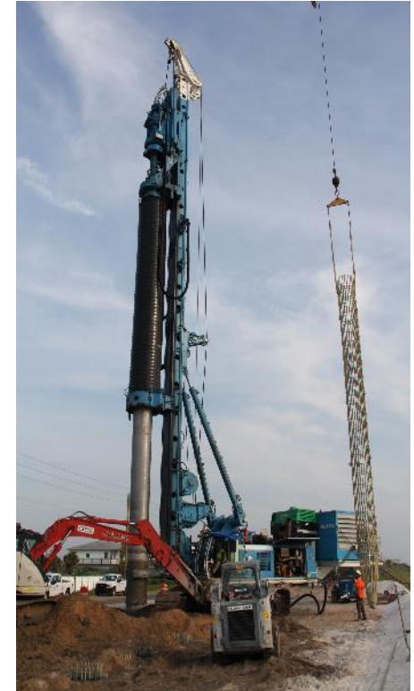
1,847 Secant-piles installed. 5,000 linear feet of pile-cap
