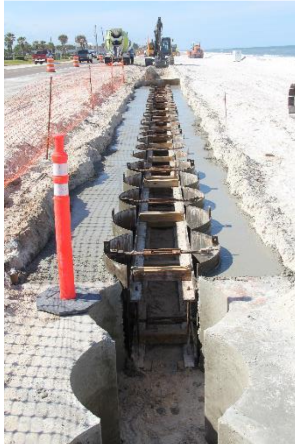
Secant-piles installed via guide wall form
