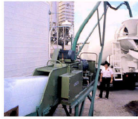
Fig. 13-6. Substituting ice for part of the mixing water will substantially lower concrete temperature. A crusher delivers finely crushed ice to a truck mixer reliably and quickly. (44236)
