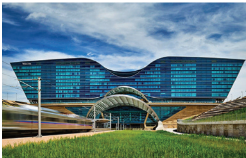
Figure 3: Denver International Hotel & Transit Center in Denver used complex mix designs including high strength, self-consolidating and lightweight concrete for the transit and hotel canopy abutments, the hotel ballroom's transfer beams and slab and the structure's sloping roof deck. Many of the walls and columns within the structure are "architecturally exposed," requiring a clean and attractive finish. Beyond being able to fulfill the project's design challenges, builders chose concrete for its fire resistance and strength.
