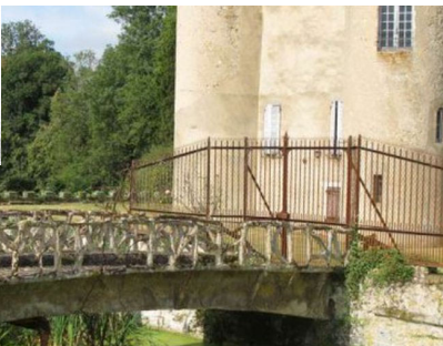
▶ Joseph Monier & the Bridge at Chazelet.
