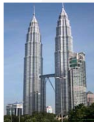
Petronas Towers, Kuala Lumpur, Malaysia - worlds deepest foundation system with piles up to 375 ft deep and a concrete raft mat measuring 15 ft thick using 17,400 yd 3 of concrete
