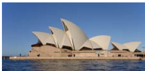
Sydney Opera House, Australia - roof structure comprises precast concrete shells; entire building sits on 588 concrete piers
