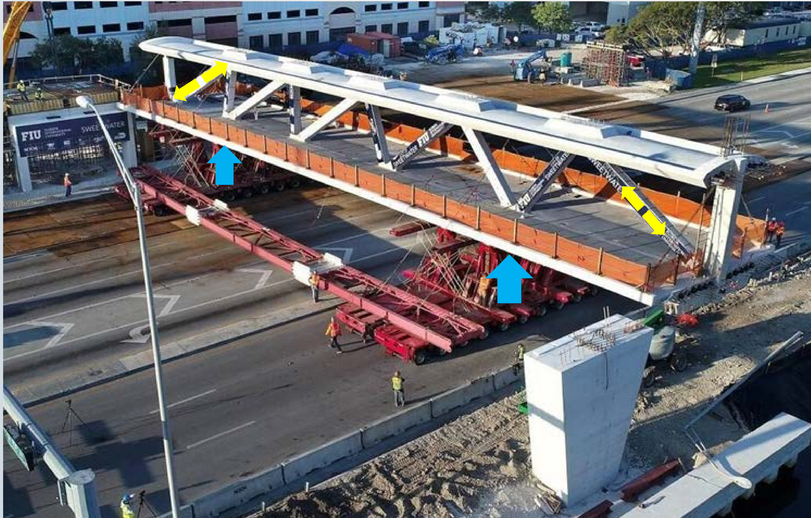
Move of Main Span into Position: March 10, 2018
