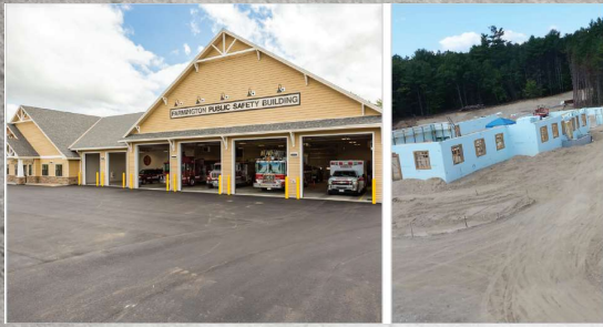
Farmington Public Safety Building, Farmington, New Hampshire
