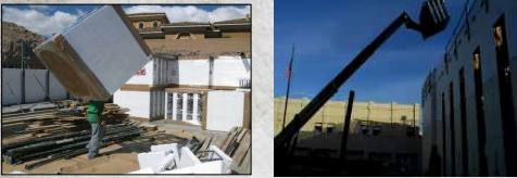
Typical ICF Bundle: (84 Lbs) at 64 Sq Ft of Wall. vs CMU equivalent (1,680 Lbs)
