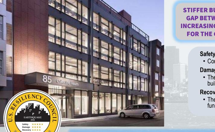
STIFFER BUILDING REDUCED REQUIRED GAP BETWEEN ADJACENT BUILDINGS, INCREASING RENTABLE SPACE THAT PAID FOR THE COST OF ADDITIONAL STEEL
