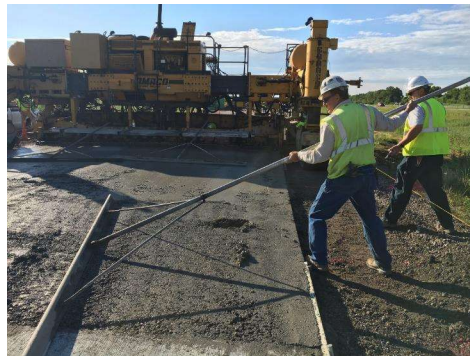
Cell 806, 5" FRC , 0.75% fibers by volume
