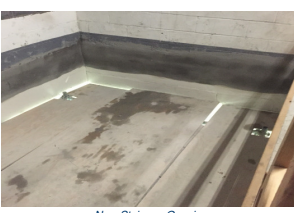
New Stairway Opening (Finished Product)
