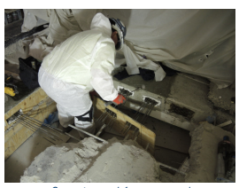
Concrete cured, forms removed
