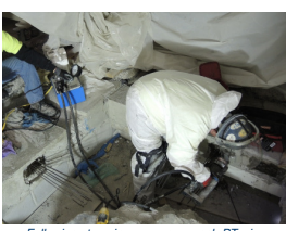
Following stressing sequence, each PT wire stressed to specified force
