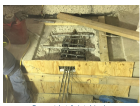
Formwork installed at slab edge
