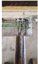
Typical End Anchor Detail
