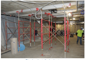
Shoring installed prior to detensioning of PT tendons
