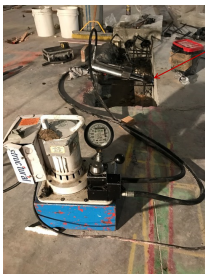
PT strand stressing (monostrand anchors)
