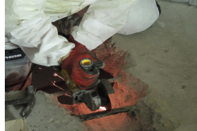
Grinder used to cut individual wires to detension tendon
