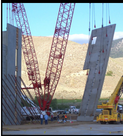
TILT UP WALL PANEL SYSTEM
