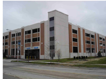
Provina St. Joe Hospital Joliet, IL
