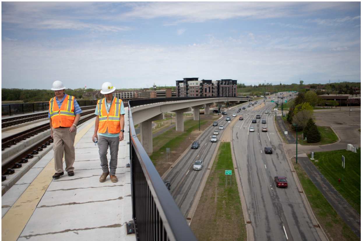
📷 Southwest Light Rail project spokesperson Trevor Roy (R) walks with a person on a bridge constructed for the light rail line during a tour. The 14.5-mile line, scheduled to open in 2027, faces cost overruns. Photo by H. Jiahong Pan/Minnesota Reformer.
