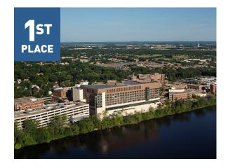
**St. Cloud Hospital East Addition**. Primarily constructed of two-way cast-in-place flat slabs, the 10 story, 450,000 ft<sup>2</sup> addition to the St. Cloud Hospital is a significant concrete structure on a complex and challenging site.
