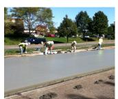
CP 12-11601 Asphalt Mill and Concrete Overlay: Valley Creek Road from Bielenberg Drive to Woodbury Drive. Aggregate Industries supplied approximately 10,000 yd³ of concrete for a 1.5 mile unbonded overlay on Valley Creek Drive in Woodbury, MN which included high early concrete to accelerate intersection openings.
