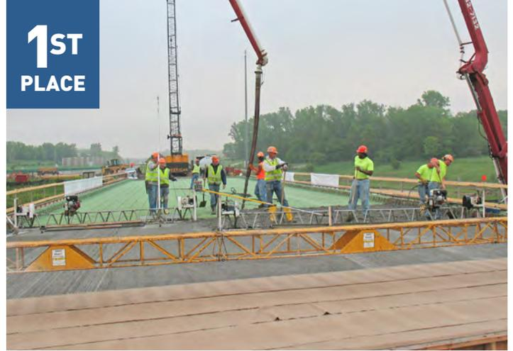
**I-694 Bridges over Trunk Highway 5.** This is the first MnDOT project that utilized a performance-based concrete mix designed solely between the contractor and concrete supplier. The bridge decks were built with innovative concrete to significantly mitigate cracking, but more importantly the bridge deck incorporated implementation of MnDOT performance-based specifications.
