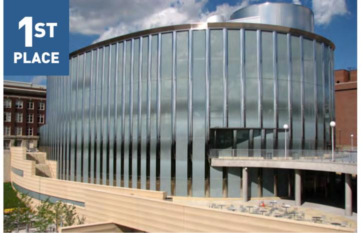
**University of Minnesota Science Teaching and Student Services.** The U of M Science Teaching and Student Services building includes architectural and structural concrete elements not seen in everyday projects, which included seamless self-consolidating columns, exposed post-tensioned slabs, pervious concrete, cast-in-place grand staircase.
