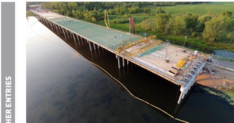
**Hwy 101 Bridge – Southwest Reconnection Project.** The project constructed a new four-lane Hwy 101 spanning the flood plain between the existing Hwy 101 Minnesota River Bridge in Shakopee and County Road 61/Flying Cloud Drive in Chanhassen. The goal was to minimize transportation disruptions caused by seasonal flooding of the Minnesota River.
