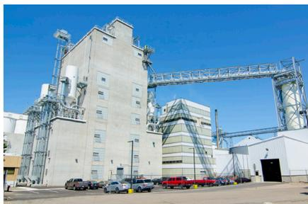
**Grain Cleaning Expansion.** General Mills constructed a new, seven-story slipformed concrete facility dedicated to processing grains to make gluten-free Cheerios. Slipform concrete meets both the sanitary and structural needs of the building.
