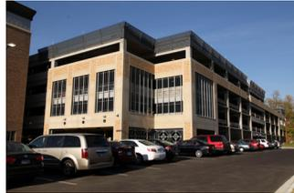
**Metropolitan State University Parking Structure.** The Metropolitan State University Parking Structure is a cast-in-place, post tension structure consisting of 773 parking spaces on 4 ½ levels with a stand-alone stair tower structure.
