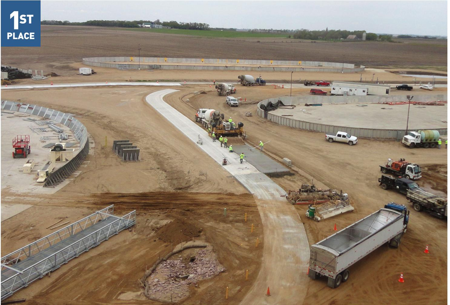
**Elevator Expansion Project.** The Pipestone project included upgrades to each component of the facility. Conventional concrete pavement was selected for the main roadway as the best option in the face of continuous stress.
