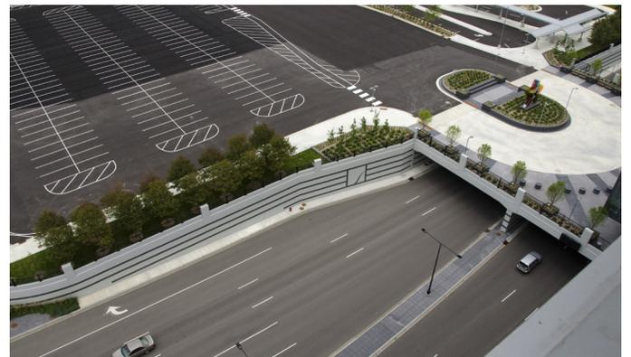
**Lindau Lane Grade Separation.** The project safely separates pedestrian and vehicular access to the Mall of America's front entrance from through traffic by lowering Lindau Lane and building a bridge across the roadway.
