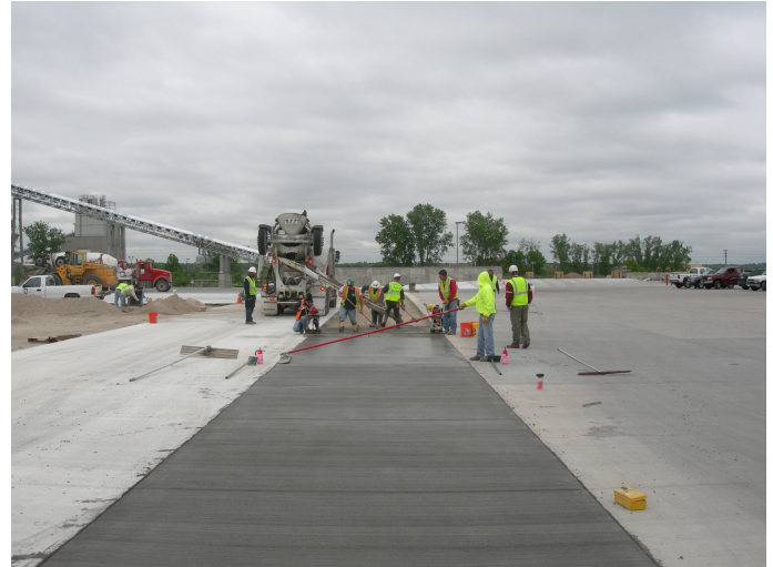
Phase III placement at AVR
