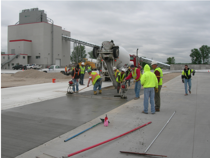
Phase III placement at AVR
