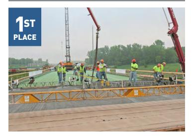
**I-694 Bridges over Trunk Highway 5.** This is the first MnDOT project that utilized a performance-based concrete mix designed solely between the contractor and concrete supplier. The bridge decks were built with innovative concrete to significantly mitigate cracking, but more importantly the bridge deck incorporated implementation of MnDOT performance-based specifications.
