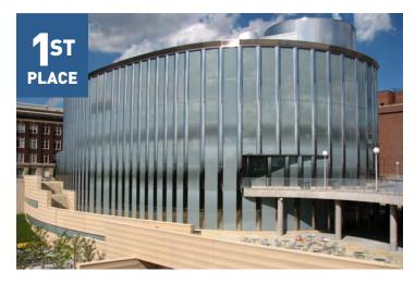
**University of Minnesota Science Teaching and Student Services.** The U of M Science Teaching and Student Services building includes architectural and structural concrete elements not seen in everyday projects, which included seamless selfconsolidating columns, exposed post-tensioned slabs, pervious concrete, cast-in-place grand staircase.
