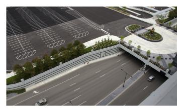
**Lindau Lane Grade Separation.** The project safely separates pedestrian and vehicular access to the Mall of America's front entrance from through traffic by lowering Lindau Lane and building a bridge across the roadway.
