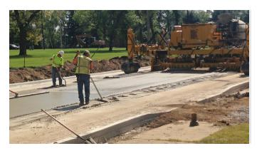
**5th Ave SW Reconstruction Project.** The City of Pipestone completed a reconstruction project on part of 5th Ave SW during the summer of 2015. Work included upgrading the underground utilities, sidewalks, curb and gutter and replacement of the existing asphalt street section with a new 6 inch concrete pavement.
