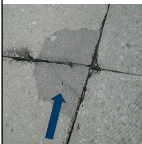
Reflective Crack at Thickness Differential
