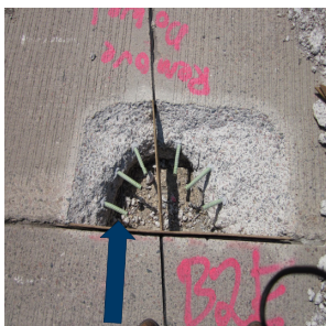
#4 epoxy coated rebar 8" long, w/4" drilled & grouted
